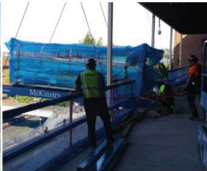
McKinstry uses multitrade racks containing multiple trade components in one prefab unit. Photo courtesy of McKinstry.
